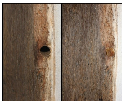
Fig.2. Small 15mm hole left behind is filled with a plug.
